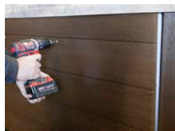
2. Unscrew and remove cabinet panel.
